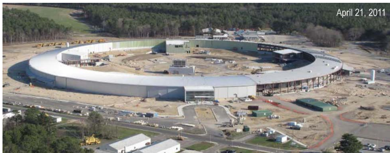
Fig 7. The NSLS-II is currently under construction at Brookhaven National Laboratory. Commissioning is scheduled to begin in 2014 and user operations in 2014. Circumference of the ring is 792 meters.
